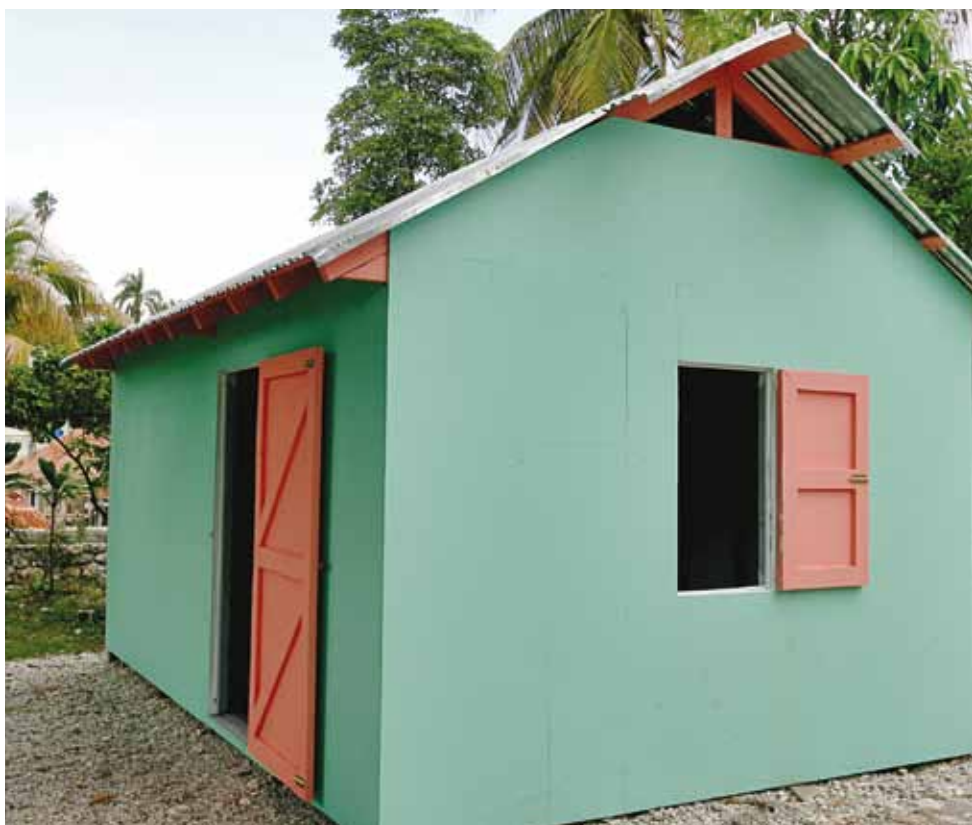
A transitional shelter provided by the Canadian Red Cross.
