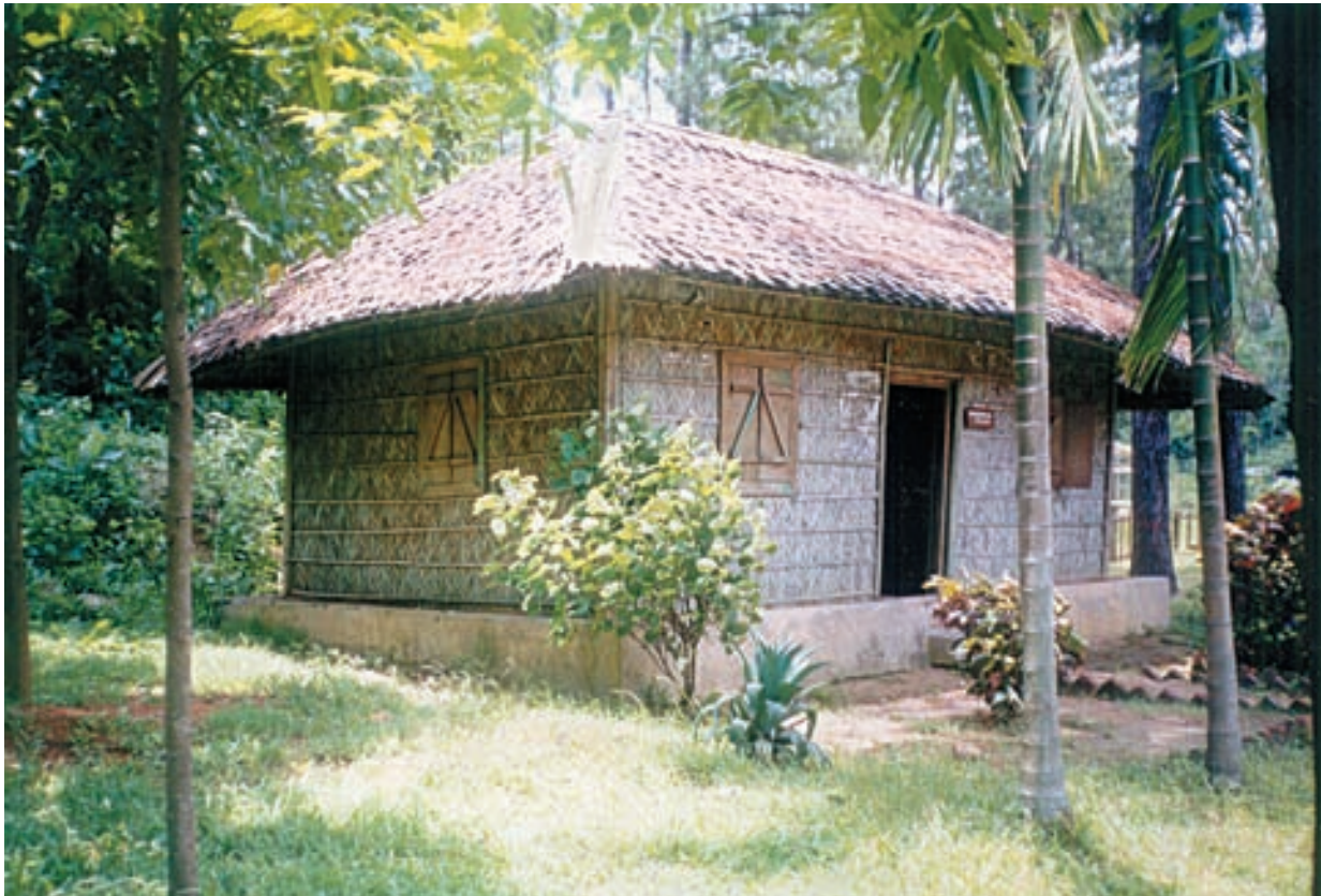
Hut built by BFRI at Chittagong - A pilot project using treated bamboo, wood, Sun-Grass etc.
