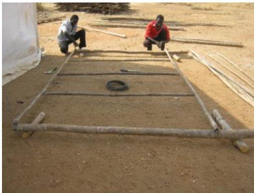
Provision of poles, bamboo and additional plastic sheeting.
