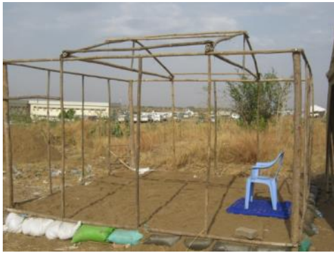
Sand bags and marrum for raising floors
