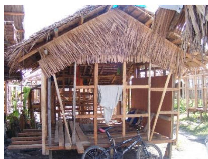
Figure 2: A shelter with coco lumber framing and nipa roofing in Tanauan, Tacloban, Philippines by NGO Green Mindanao. (Photo: K. Balson, Building Research Establishment Ltd.)
