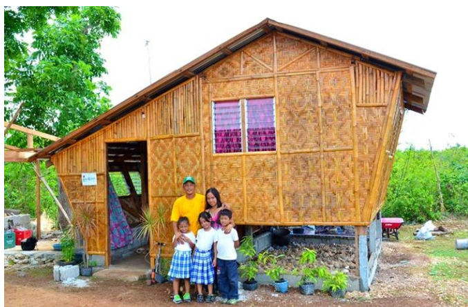
Figure 3: Shelter with amakan wall cladding, YPDR PAH Joint Housing Program, Bantayan Island, Philippines. (Photo: Joseph Ferris III, YPDR)
