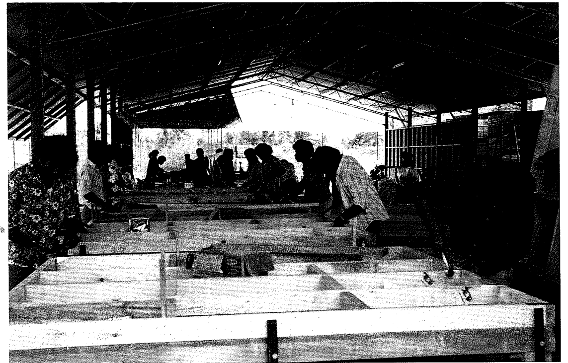
Figure 12 Factory prefabrication of Tongan housing
