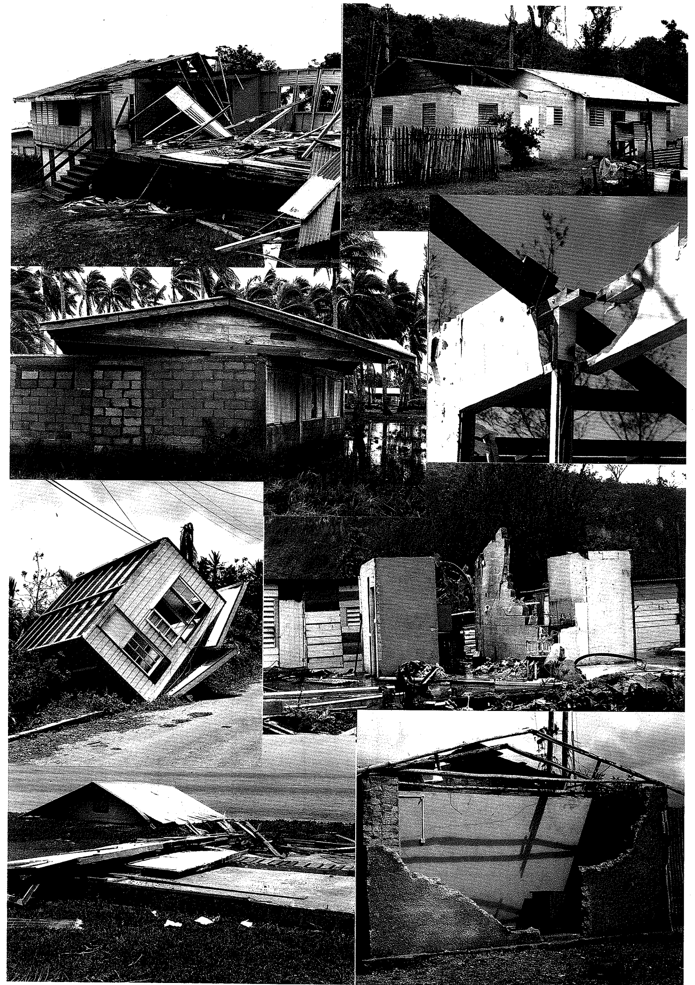
Figure 2 Examples of damage to buildings by cyclones
