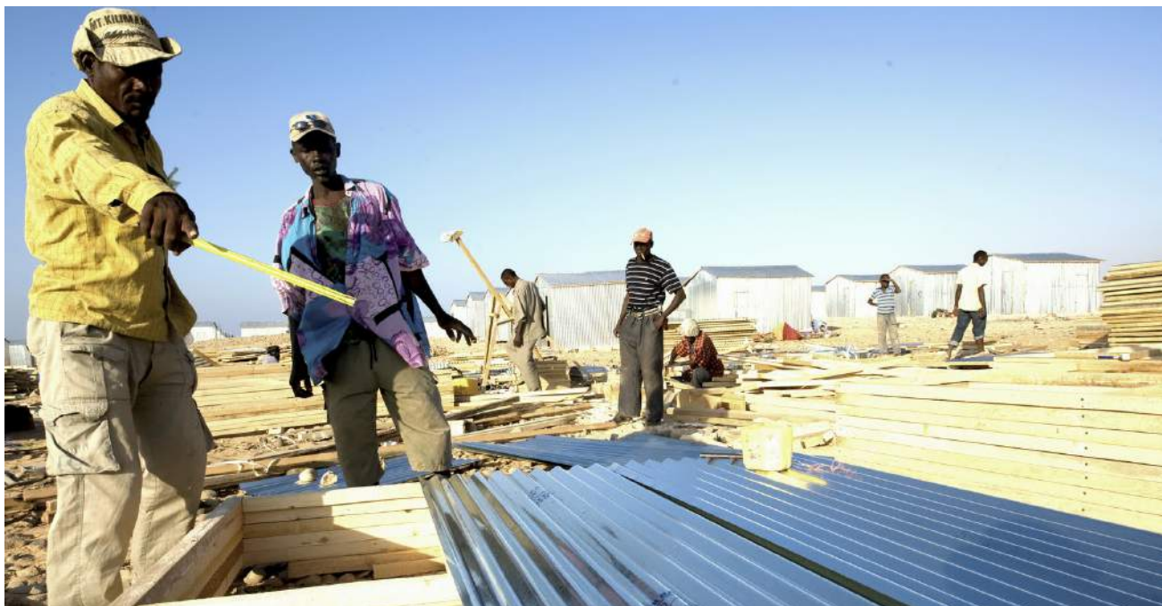
Shelter construction in Puntland, Somalia. Photo: C. Jepsen/NRC
