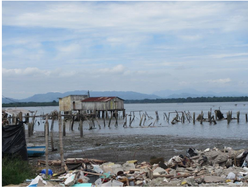
Figure 12 – Buildings built near-shore in Chamanga founded on timber and concrete piles manually placed down to about 1-1.5m deep. The piles seen were previously used for one to three storey buildings.
