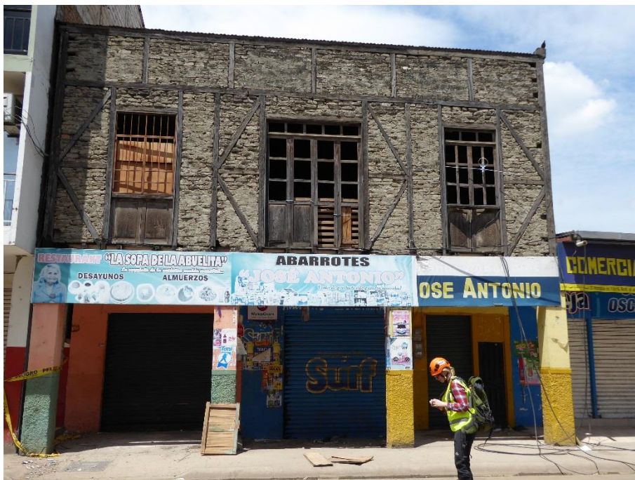
Figure 3 – Timber frame with masonry infill
