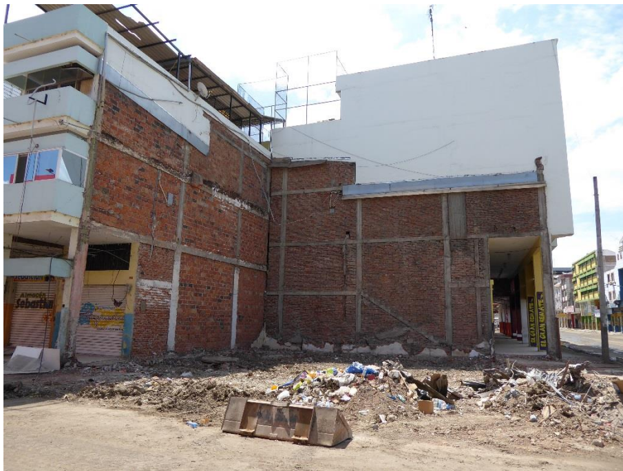
Figure 1 – Reinforced concrete structure with masonry infill walls
