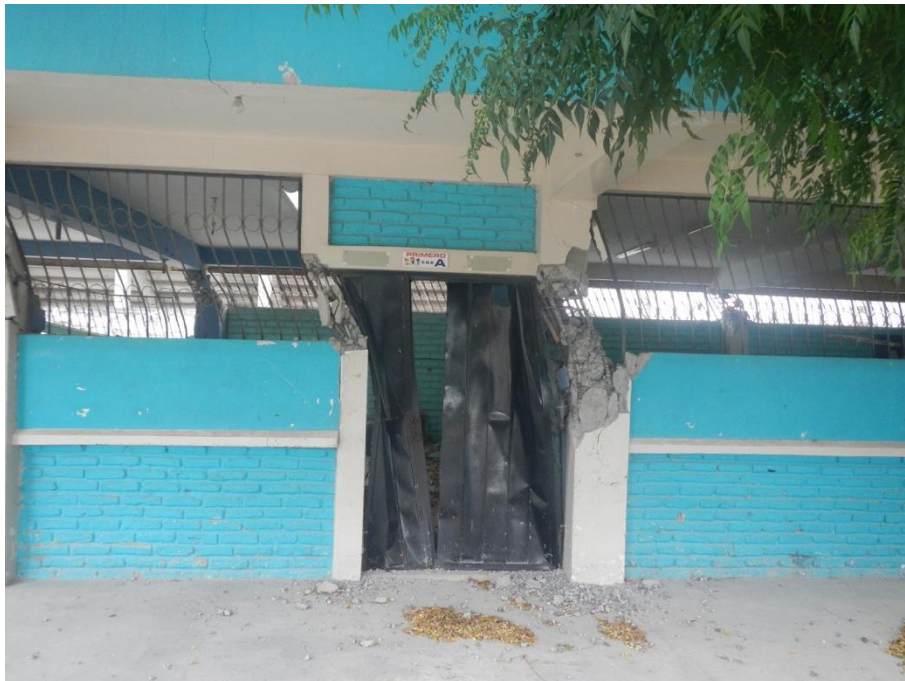
Figure 14 – Short columns at a school in Pedernales
