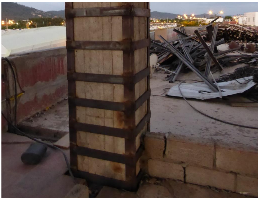
Figure 7 – Site welded steel plates for column strengthening in Portoviejo airport
