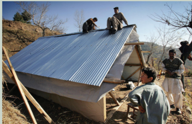
Constructing demonstration shelter, 2005.
