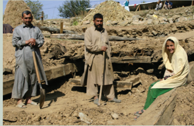
Most local houses pancaked, extensive timber salvaged.
