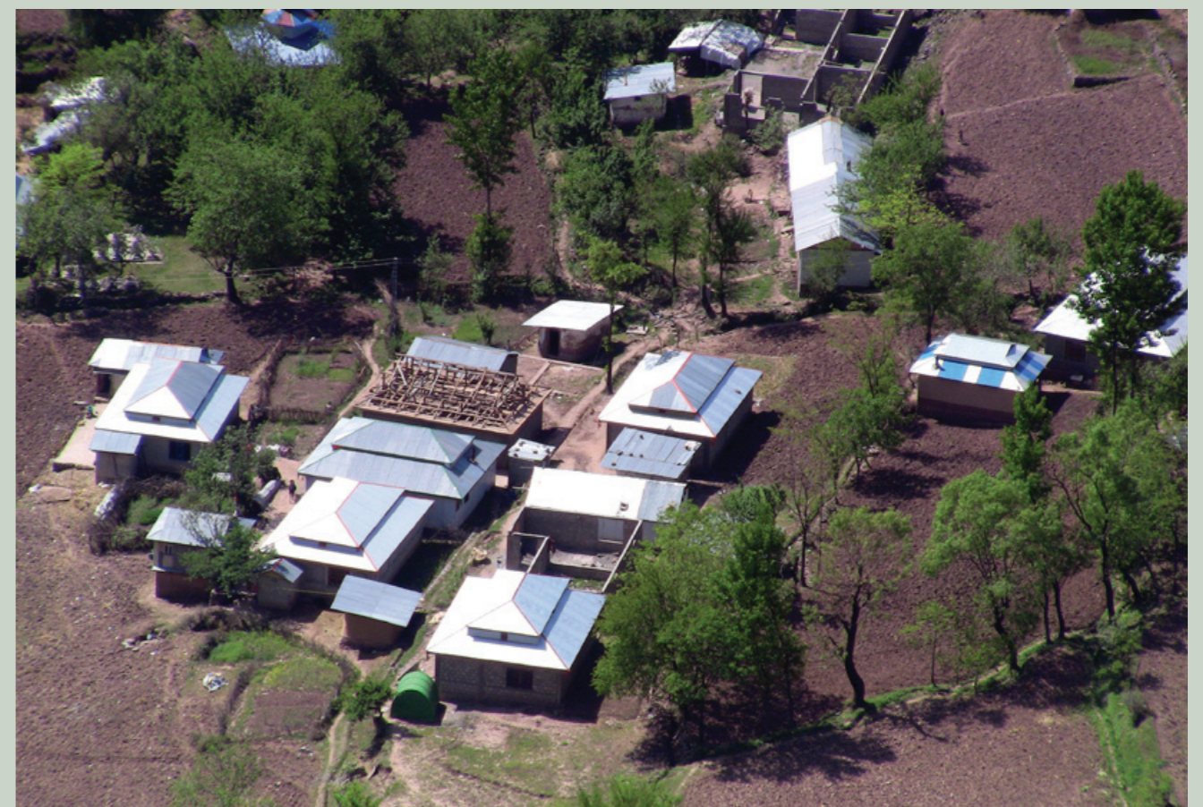
New typical housing and settlement pattern in the earthquake affected area. Note change to lighter roofs, and individual houses.
