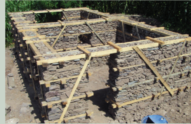
Timber reinforced masonry construction.
