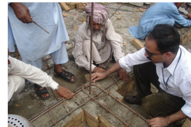
Ahsan explaining reinforcement details with masons.
