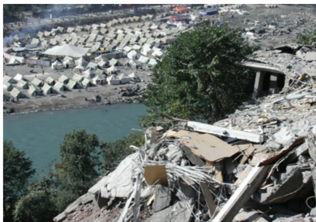
Muzaffarabad in 2005, extensive damage and displaced families.
