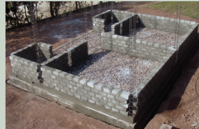
Confined masonry block construction, demonstration house.
