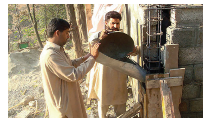
Engineer (left), learning practical concreting from mason (right).
