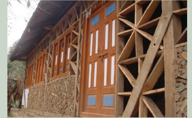
Masonry infilled timber frame, local techniques regenerated.
