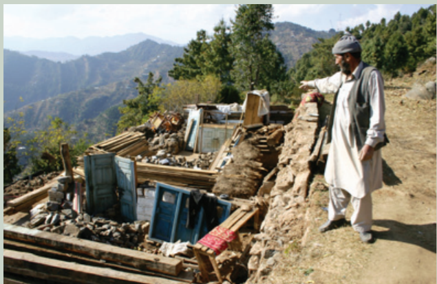
Narrow terraces, many houses include retaining walls.
